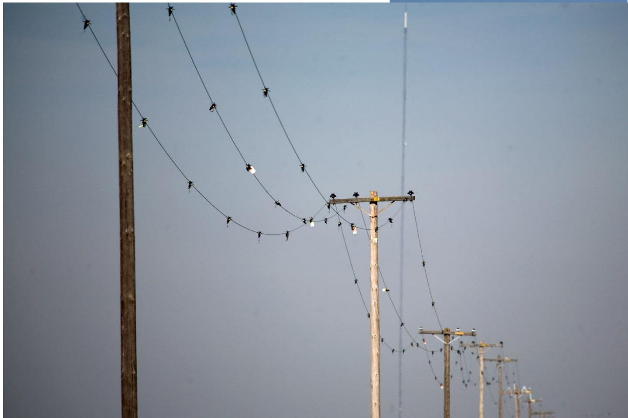
Figure 24B. Several years after deployment the line markers used to experimentally test whether line collisions could be reduced for sandhill crane and other birds (Yee 2007) were broken, twisted and missing due to exposure to sun, rain and wind. Durability is an issue. Photo by Shawn Smallwood.
