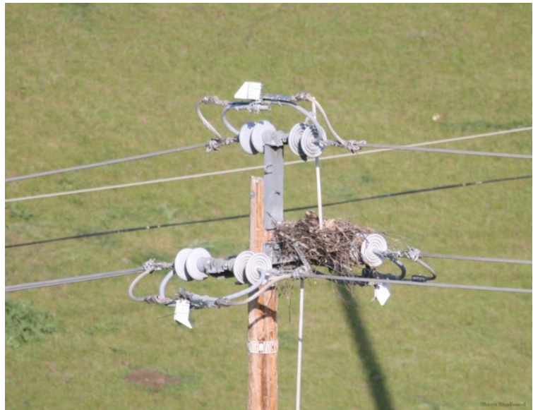
Figure 11. Red-tailed hawk nests on a distribution pole. Nest material can sometimes form a circuit between phased elements of the pole, thereby endangering the nesting birds. Photo by Shawn Smallwood.
