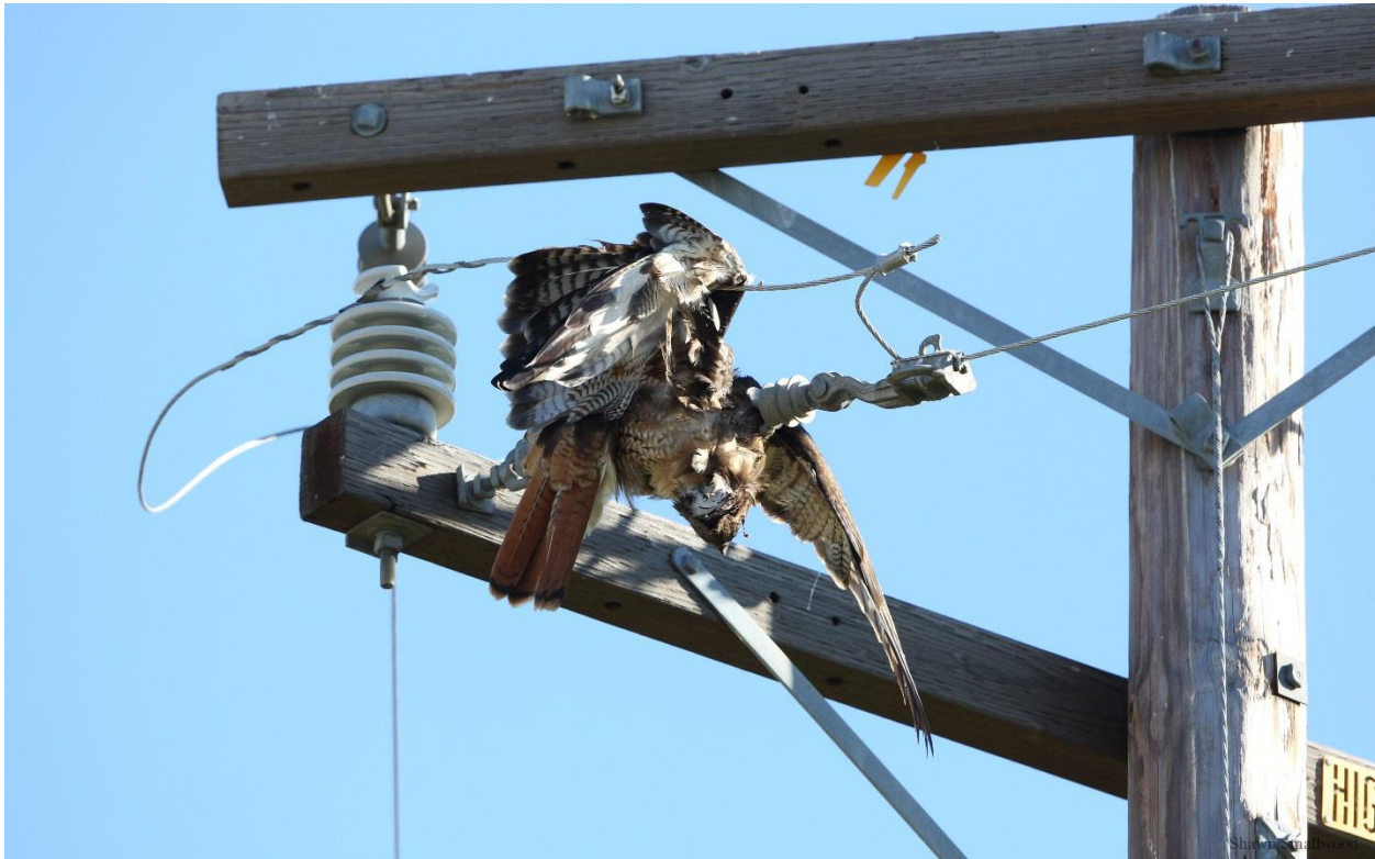
Figure 5. Red-tailed hawk electrocuted on a distribution pole servicing cell towers in Contra Costa County. Photo by Shawn Smallwood.
