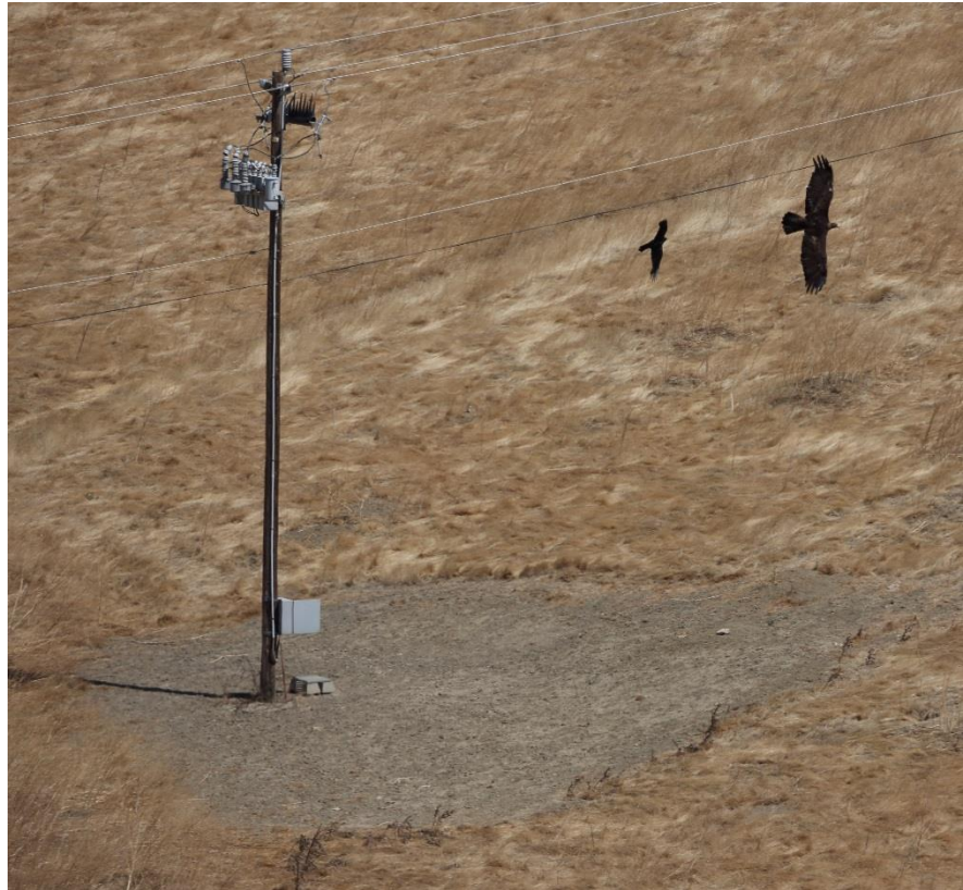
Figure 8. A golden eagle is mobbed by a common raven near distribution lines, which increases the risk of line collision. Note the bare ground around the equipment-bearing pole, which is intended to reduce the risk of fire destroying the pole as well as fire spreading from the pole should electrocuted birds fall to the ground. Note, also, the perch guard installed to discourage birds from perching on the pole. Photo by Shawn Smallwood.
